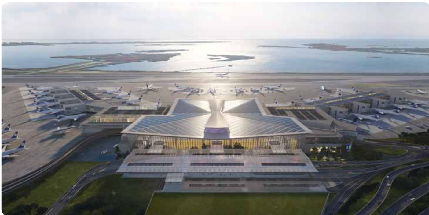
The first phase of New Terminal 1 at JFK is planned to open in June 2026 (all photos: New Terminal 1).
